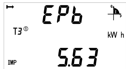
Current forward active energy on B phase
