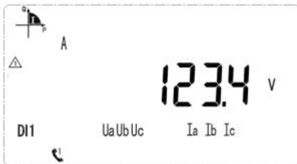
Voltage on A phase is 123.4V
